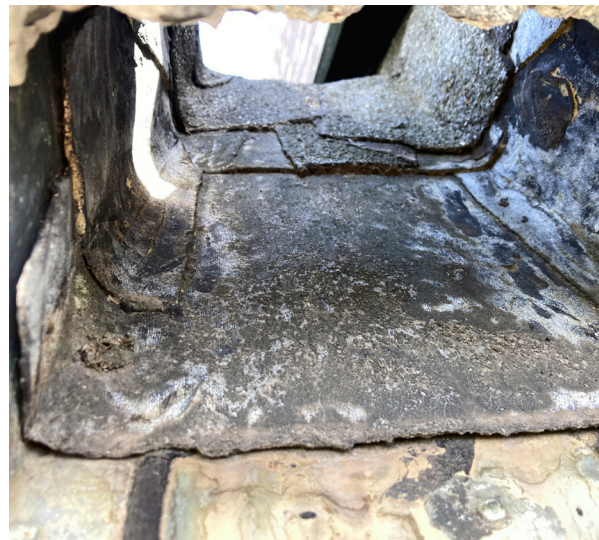
FIGURE 11: Bituminous membrane in water channel
