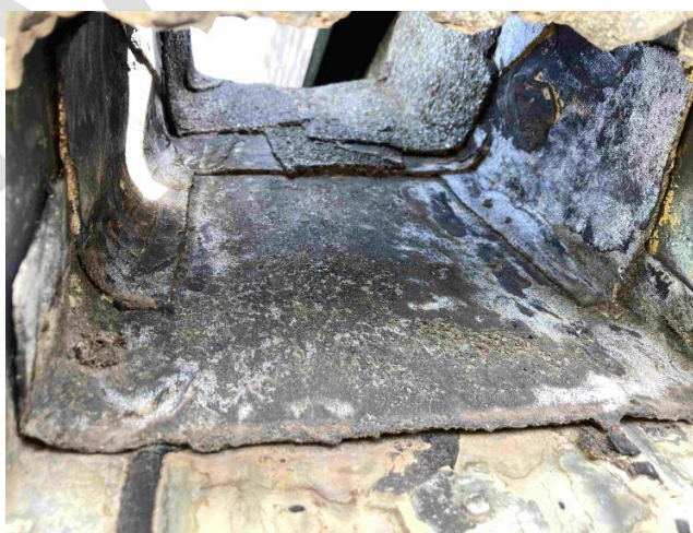
Figure 11: Bituminous membrane in water channel
