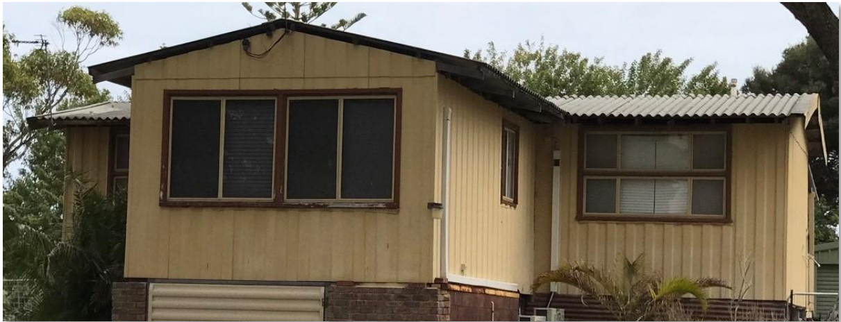
Figure 14: Residence with multiple AC structural components
