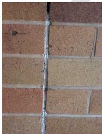
Figure 2: Sealant in wall expansion joint
